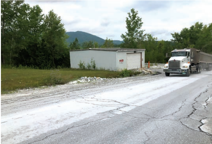
Pittsford Fire Department substation currently resides on the Omya site located along the haul truck road
